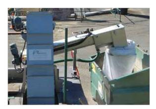
All Aqualitec Corp. bar screen are totally enclosed. To keep the odor control, the washer compactor is provided with a bagger system.
