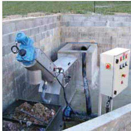
To retrofit any kind of structure, the Spiraltec can be built in tank with an integrated bypass.
